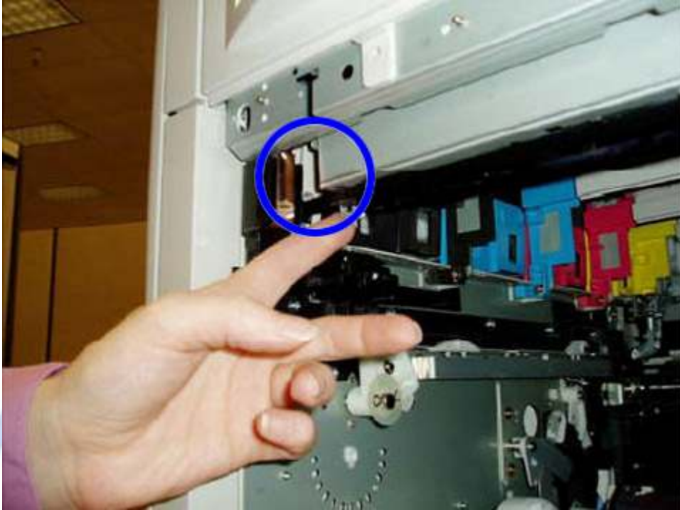
Figure 2: Actuator arm hooked into place
