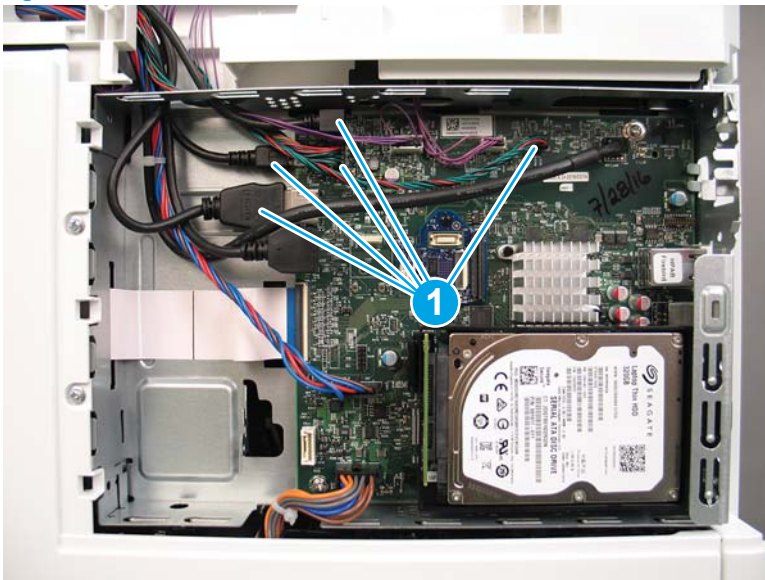
Figure 1-1918 Disconnect five connectors
