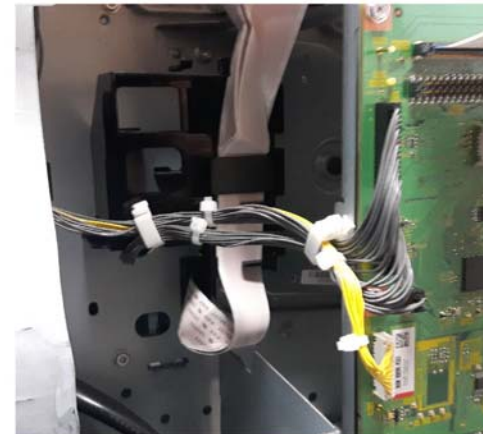
Figure 5 Wire harness removal
