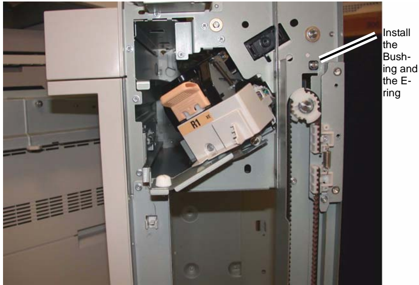
Figure 16 Installing the Bushing and E-ring
