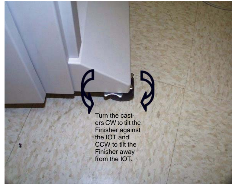
Figure 2 Leveling the Finisher
